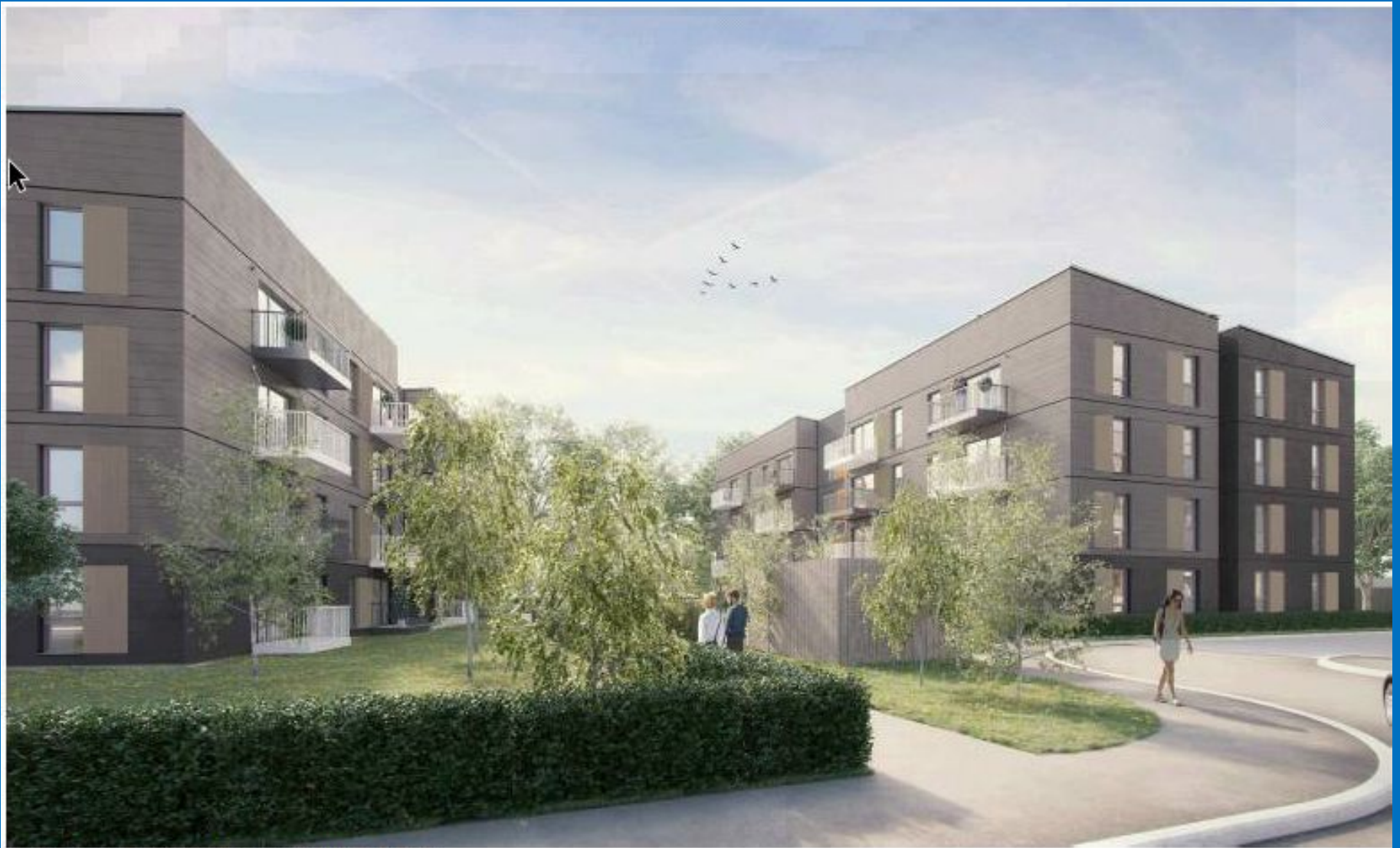
View from site entrance looking west towards blocks 2 and 3
